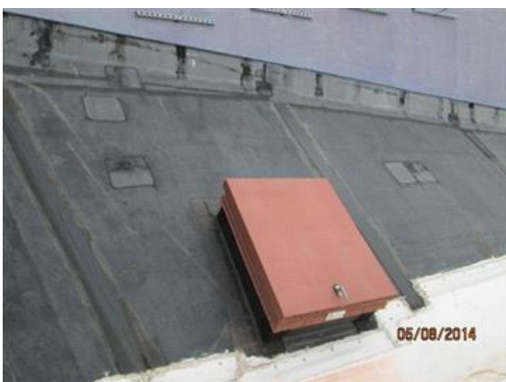
Hatchway into larger and higher parapet section.
