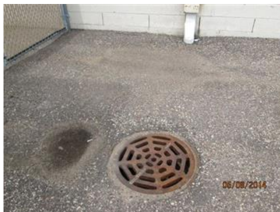
Catch basins on the property take rainwater from the roof through downspouts and underground into the catch basins.
