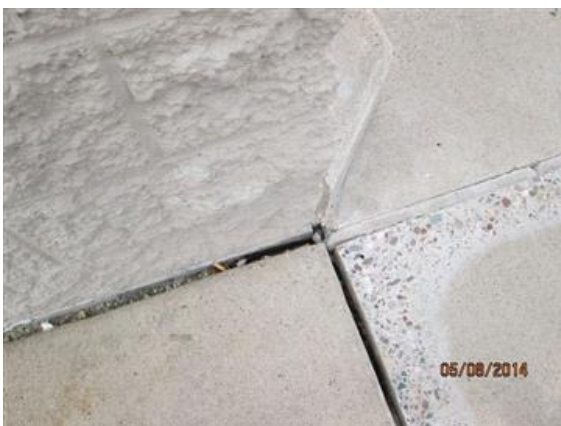
Movement of sidewalks at foundation.
