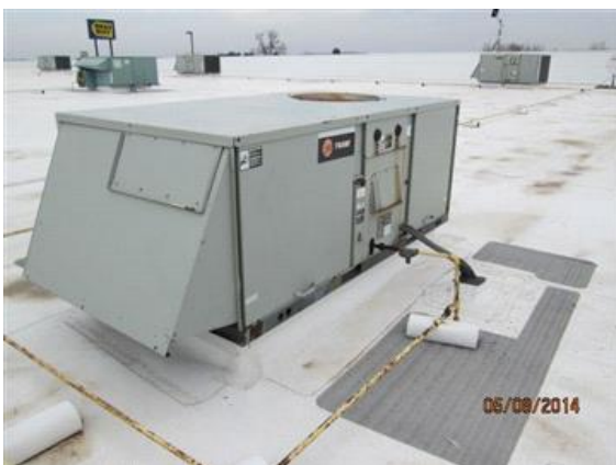
Roof Top Unit - Typical discharge directly into the space below with minimal distribution.
