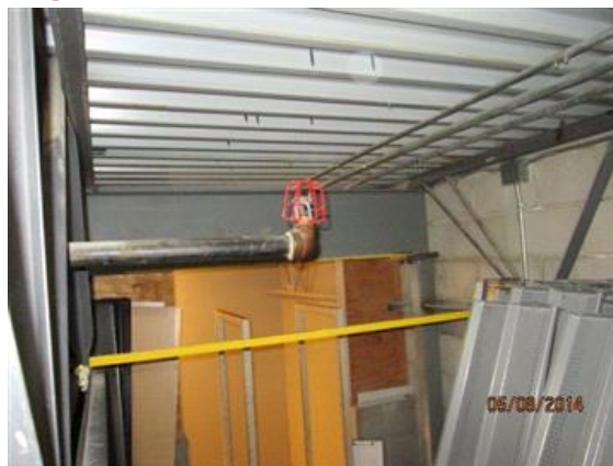
Fire protection system at roof metal decking.
