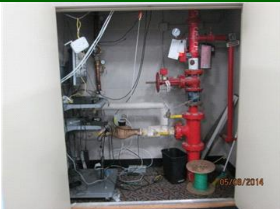
Fire protection and water service closet.
