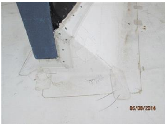
Membrane flashing at parapet wall.
