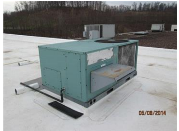
Roof Top Unit accommodates both heating and cooling.
