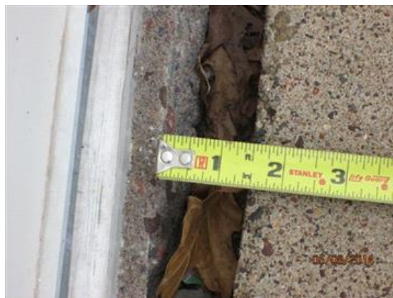
Sidewalk has pulled away 1.5" on the east side of the building.
