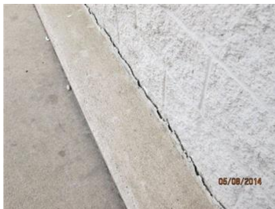
Open joint at foundation wall.
