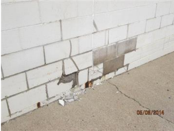
Deteriorated concrete block face.
