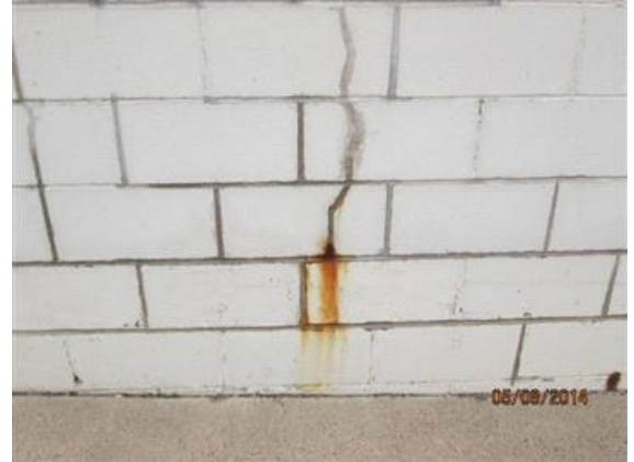
Concrete block vertical crack with rust.
