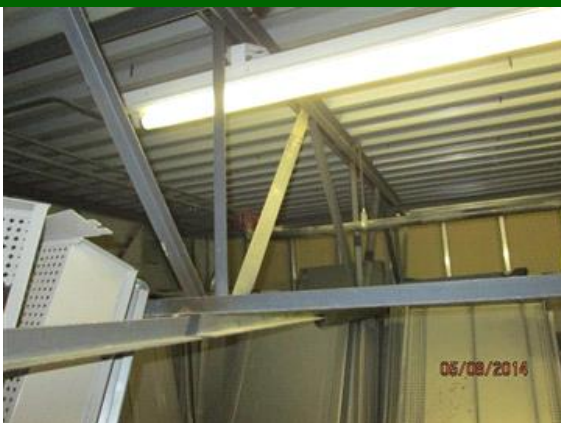
Detail of joist and decking.
