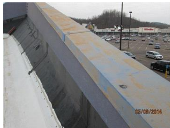
North side galvanized top cap flashing that is showing signs of rust.
