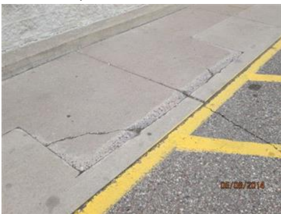
Sidewalk area that has been ground down to eliminate a tripping hazard.
