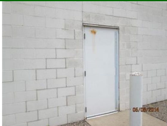
Exterior service door - note spot of rust at top of door.
