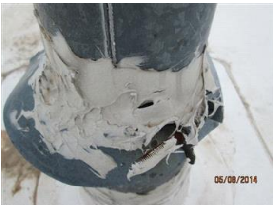
Open hole in caulking at vent pipe.
