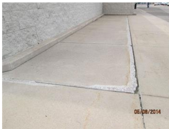
Sidewalk at front of store showing signs of settlement. Has edges ground down.
