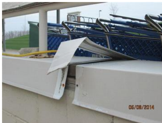
Top cap is damaged on the loading dock retaining wall.
