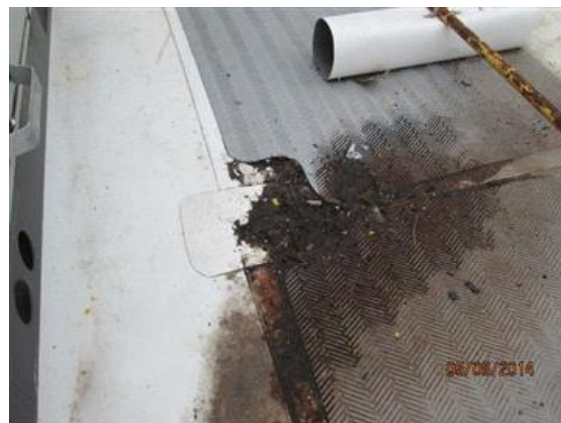
Dirt has settled in the ponding area.
