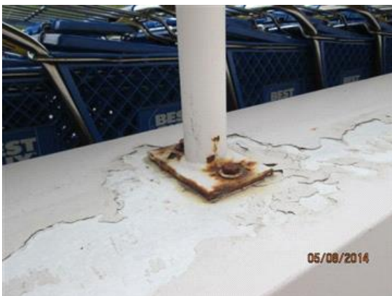
Rusted bolted connection of railing on top of loading dock wall.
