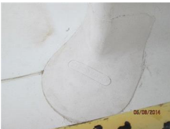
Membrane roof joint. Typical, in good condition.
