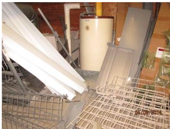
Access to water heater above ceiling space was blocked by stored materials.
