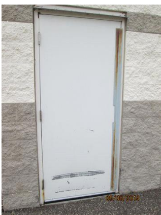
Service door with scratch in the bottom of door and a small spot of rust at base of frame.
