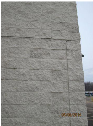
Vertical crack in concrete block at corner.
