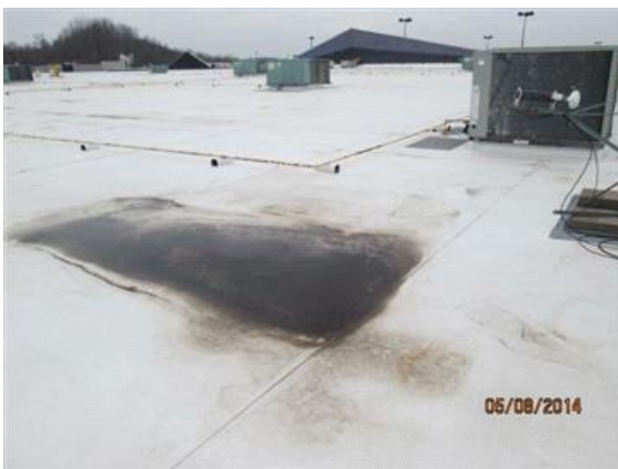
Area of ponding on the roof.
