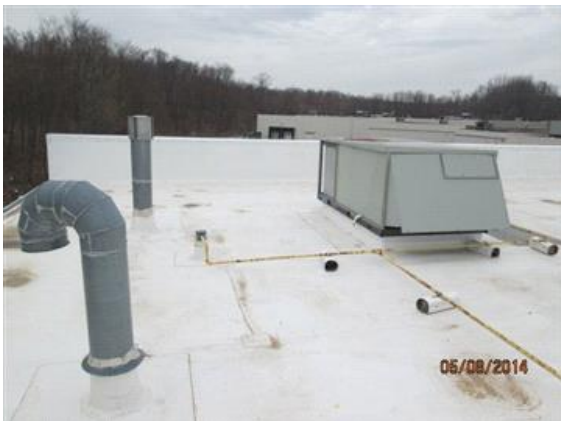
Roof Top Unit and exhaust venting.
