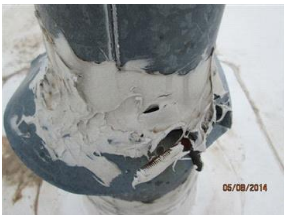
Open hole in caulking at vent pipe.
