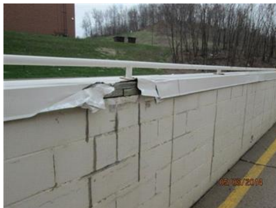
Retaining wall damaged top cap and block mortar joints in need of painting.
