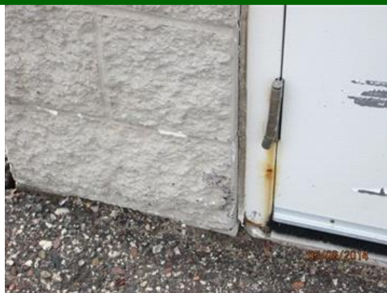
Rust at bottom of service door.
