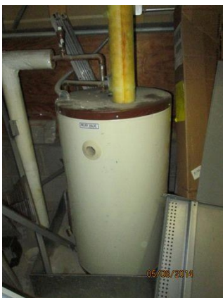
Water heater above ceiling space.
