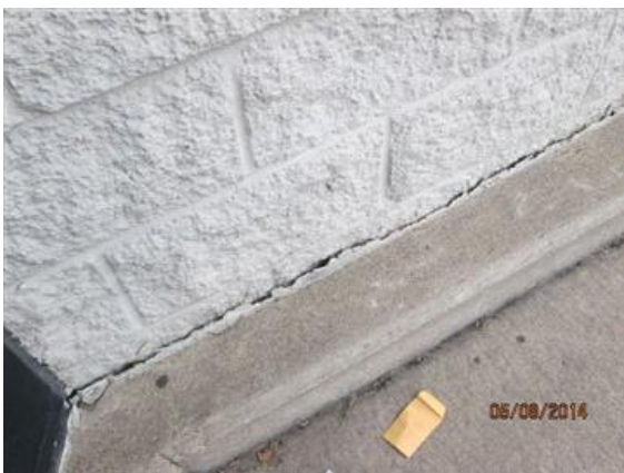
Open joint at foundation wall.
