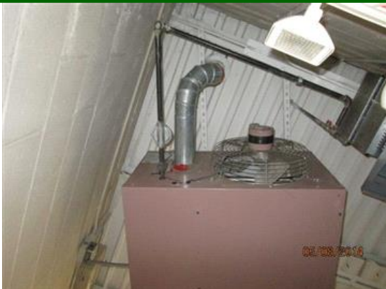
Gas fired unit heater ventilation through roof.
