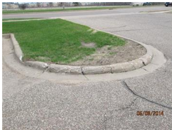
Curbing at southeast driveway. Note the 'drive over' area of dead grass.
