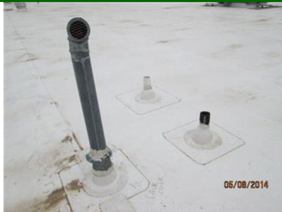
Typical roof penetrations.
