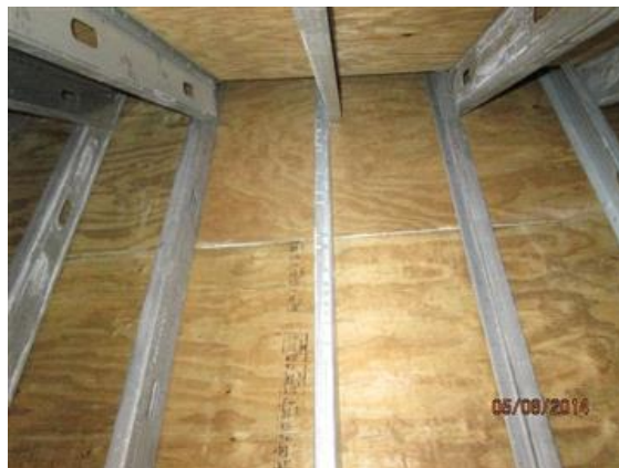
Framing of front parapet wall - metal studs and plywood.
