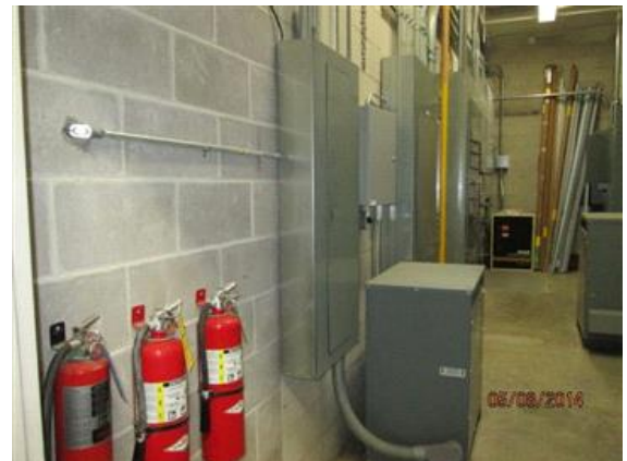
Main electrical service room with panels and main disconnect.
