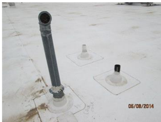
Typical roof penetrations.
