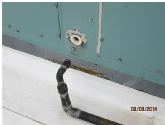
RTU - 7 condensate line is disconnected from unit.
