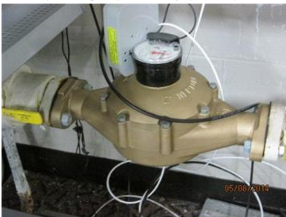
Water service meter located near the fire protection riser in closet off of retail floor.
